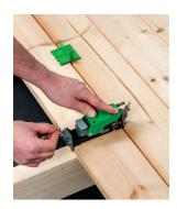
3. Place a screw in each installation hole. Use the spacers for the correct distance between the boards.
