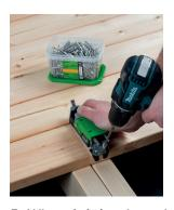
5. When joining boards: Install an additional joist at the joint.
