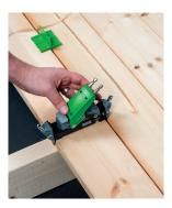
2. Place the tool over the joist and clamp the tool to the board.
