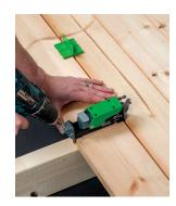
4. Screw the ESSVE HDS screw using the HDS bit with red marking. Always start with the outermost screw.
